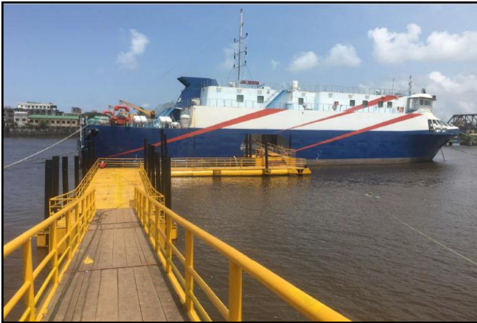
Constructed floating jetty at Daman
