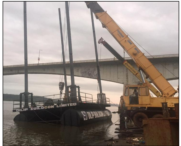
soil investigation jack up launching after construction
