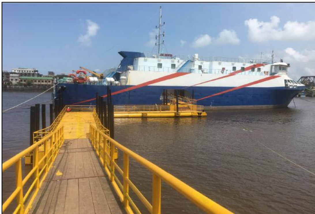
Floating Jetty Design and Actual Photo at Daman
